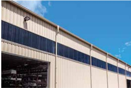
***A row of clear panels just below the roofline draw in natural light and help reduce the amount of electricity needed to light the building.***
