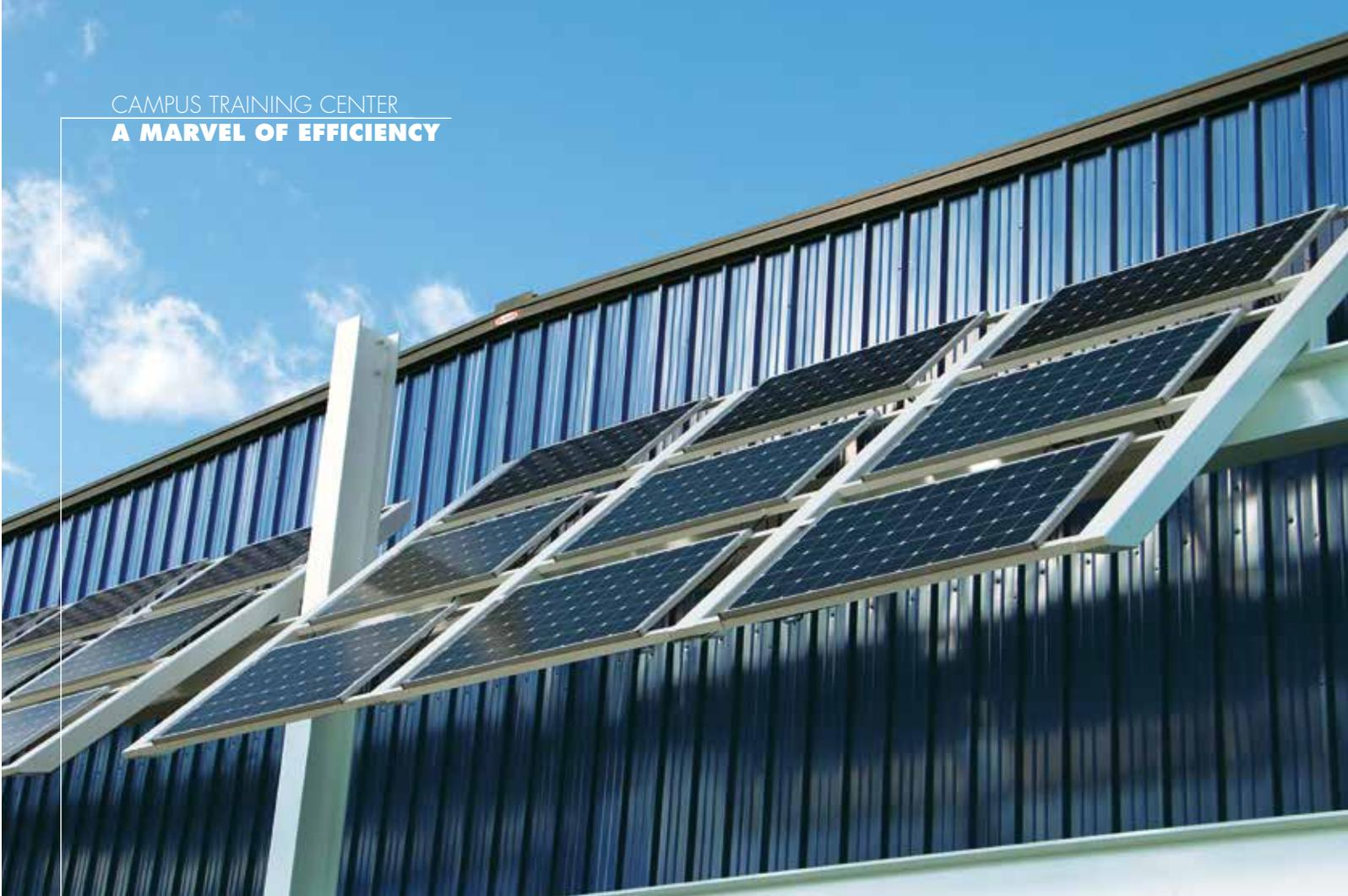
*Iowa Lakes Community College incorporates many features to enhance both mechanical and energy efficiency, including the SunLite Strip® daylighting system and a photovoltaic (solar) system to reduce electrical costs.*
